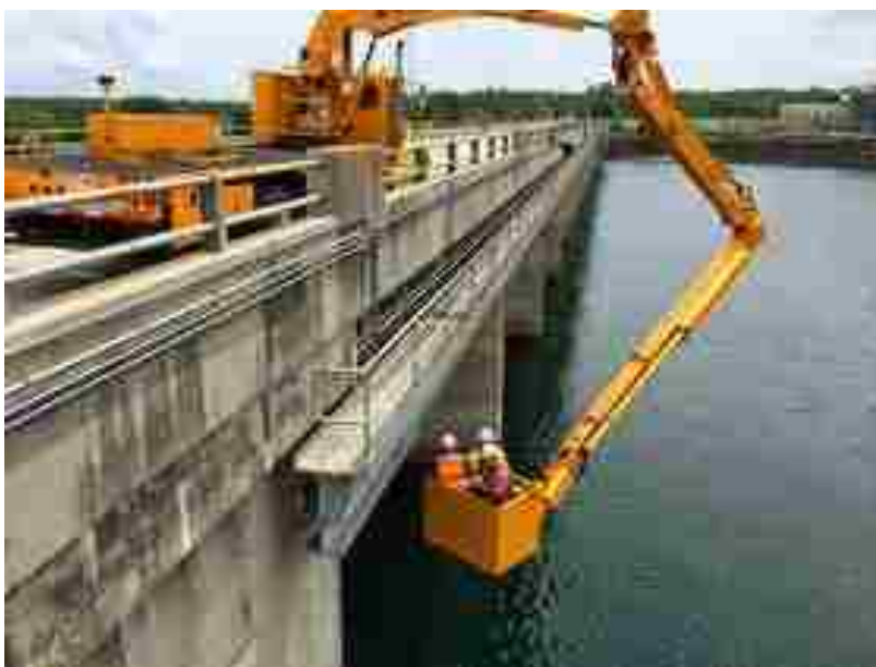
Figure 1.1: Typical damage assessment by the inspection team
